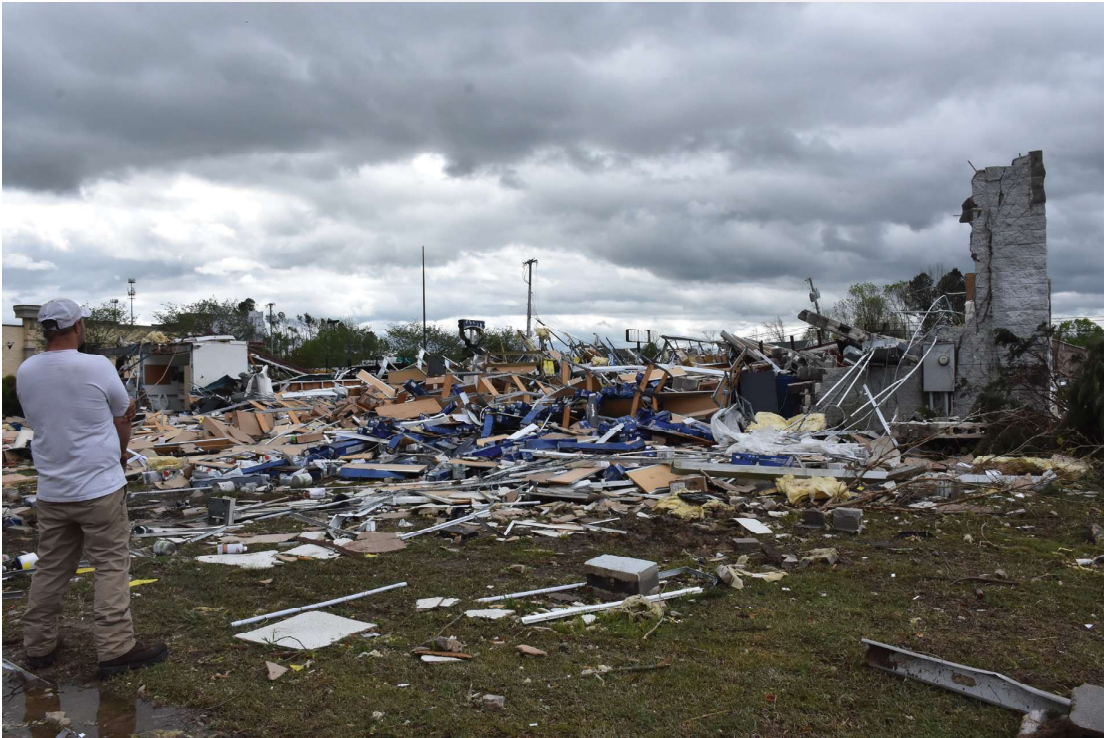
Damage to the AutoZone store on East Brainerd Road in Chattanooga, 2020.
