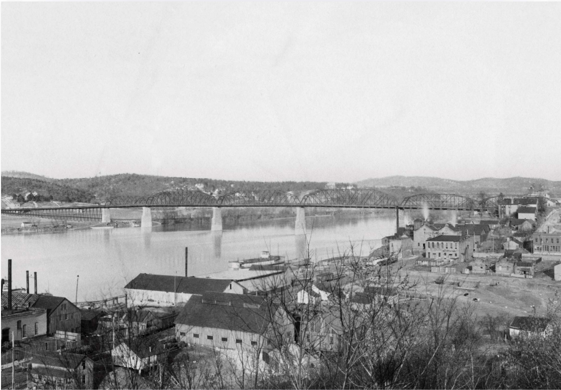
Above: The construction of the Walnut Street Bridge, dated June 16, 1890, photograph by Steven Clay Dodge.
